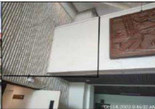
PABX, Cashier, & Front Office
