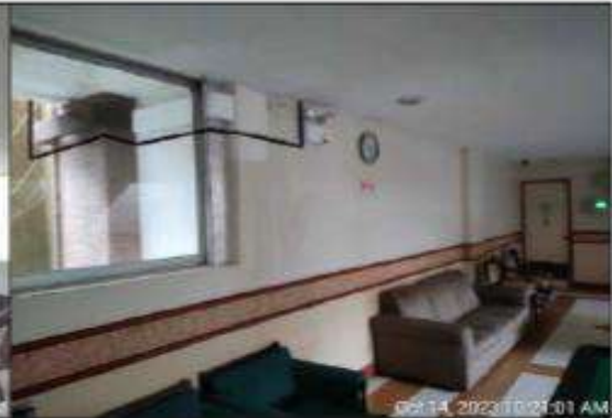
Basement Lobby to EE Room, & Hallway
