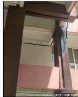
Back of 2nd Floor Lobby, & Room 201
