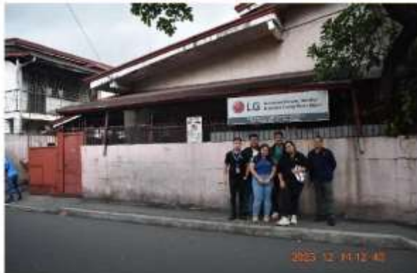
The Site – Jholan Airconditioning Services .
